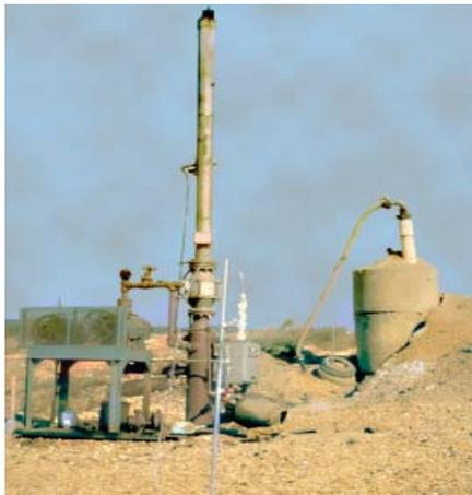
Devices used to combust gas at modern landfills have more than a 99 percent destruction efficiency for methane and a 98 percent rate for other gases.
