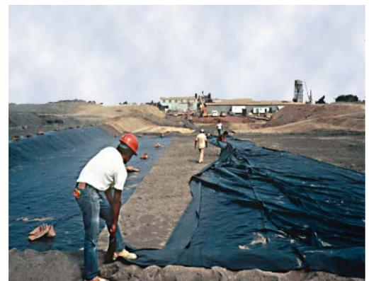
Synthetic materials can be used as landfill liners to prevent contamination of groundwater resources.
