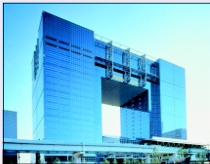
Telecom Centre Building. Photo: WTA
