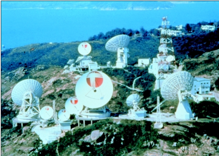
The Stanley earth station. Photo: Hongkong Telecom
