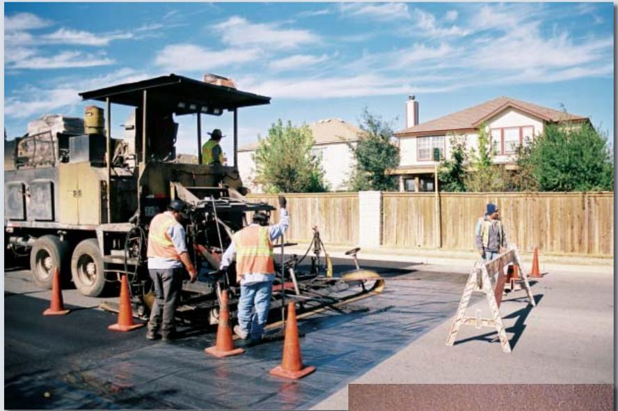
Above: Viking Construction crew uses an Akzo Nobel machine to apply micro surfacing on an arterial on the outskirts of San Antonio.
