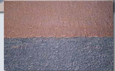
Right: As water in slurry mixture evaporates, micro surface color changes from brick-red to black.
