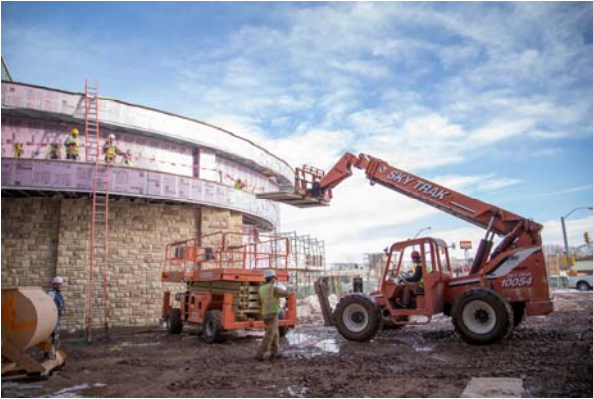
Construction on the Legacy Hall Jan. 15, 2014
