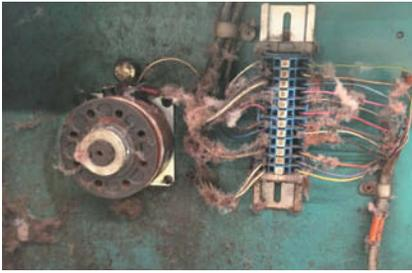
**Lint build-up inside the control panel can cause erroneous signals and potentially catch fire if ignited by a spark.**
