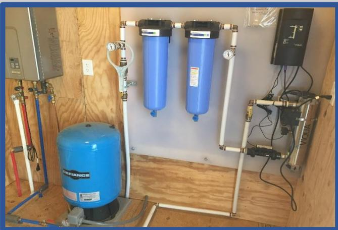
Sample post-tank water treatment system including a sediment filter, carbon filter and ultraviolet light.
