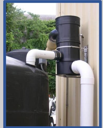
Sample self-cleaning rainwater harvesting pre-tank filter
