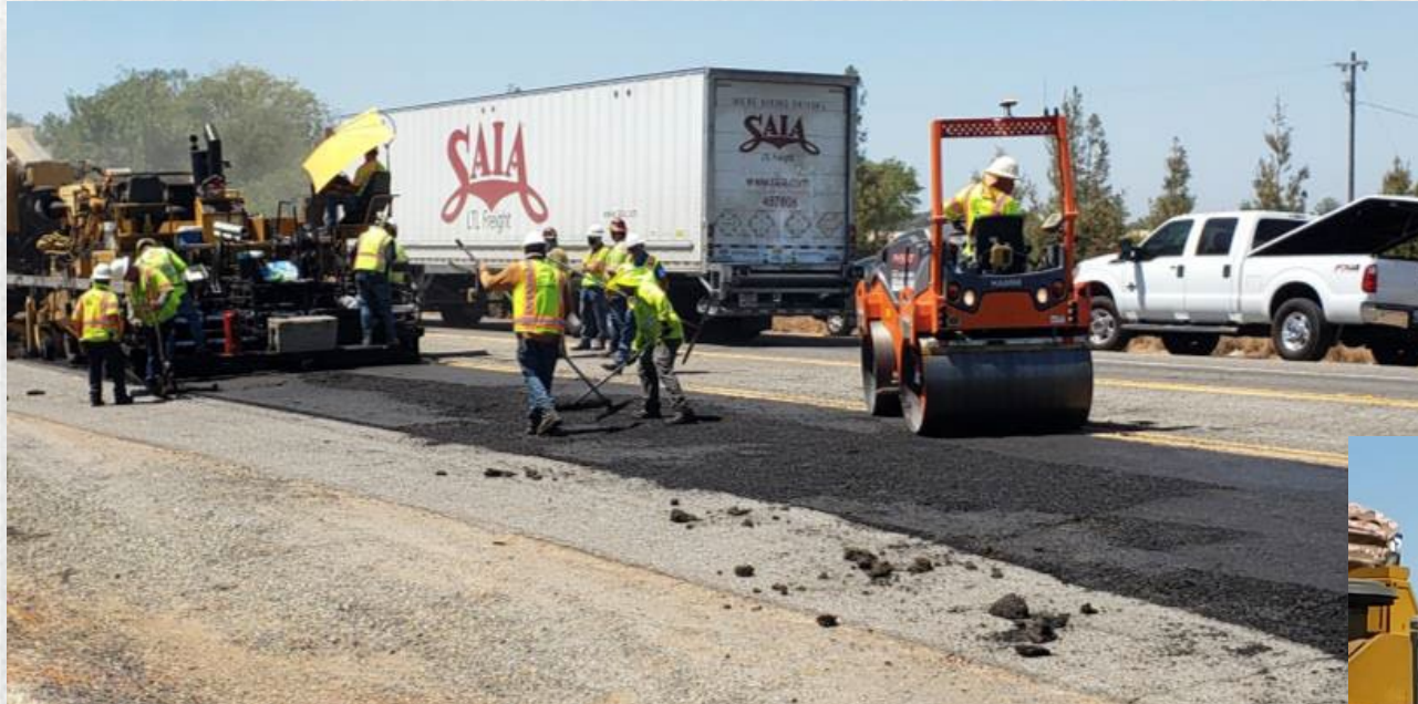
Broadcasting (handwork) behind paver
