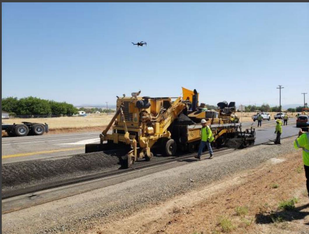
Pickup and Paving
