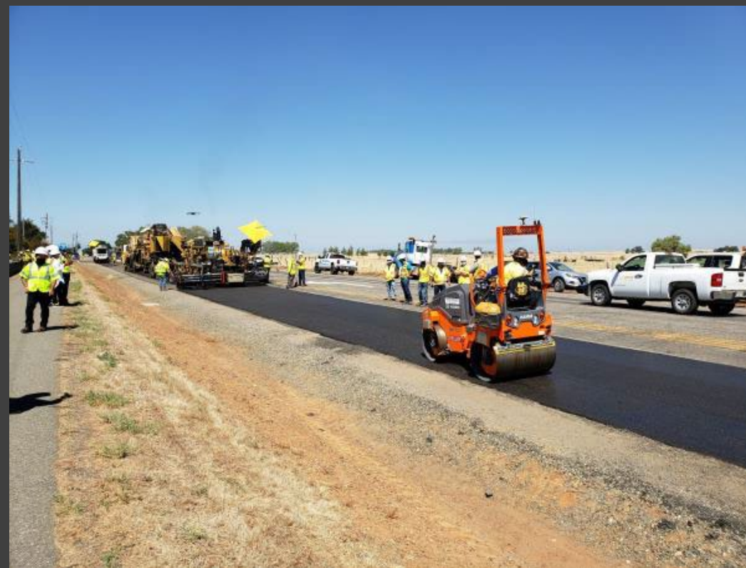
Rolling and Compaction
