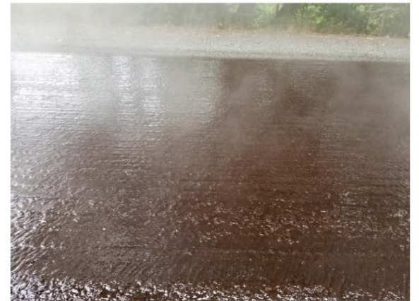
Freshly applied emulsion
