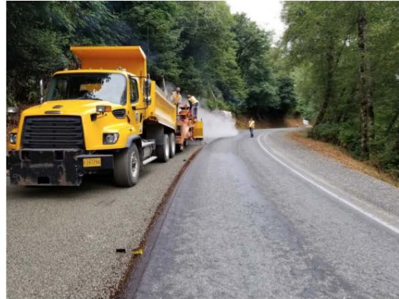
Chip seal in process
