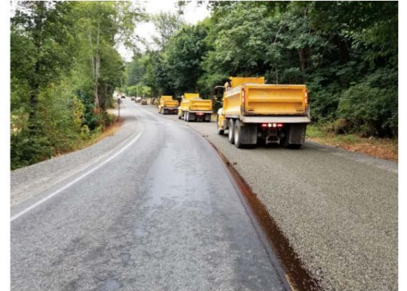
Chip seal in process
