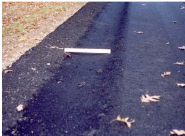
BITUMINOUS GUTTER DETAIL
