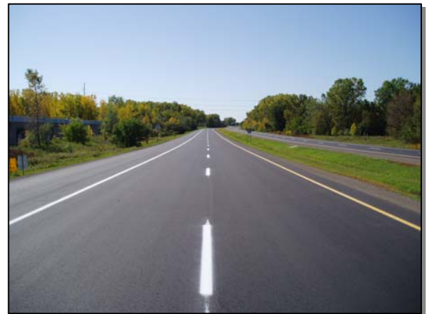
Figure 2. Ramsey CSAH 88 Completed.
