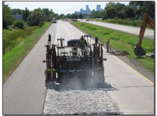
Figure 1. Rubblizing Ramsey CSAH 88.
