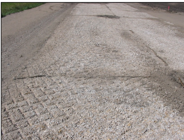
Rubblizing the deteriorated pcc on CSAH 16 prior to overlay.
