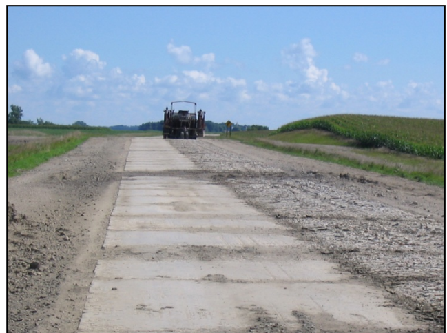
Rubblizing the deteriorated pcc on CSAH 16 prior to overlay.
