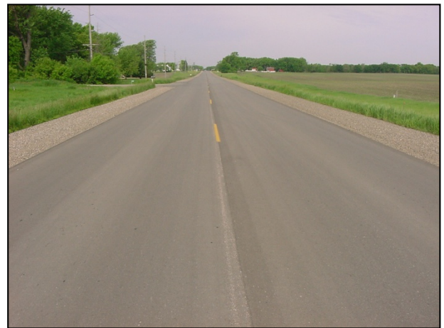
CSAH 16 prior to final 1½-inch wear course.
