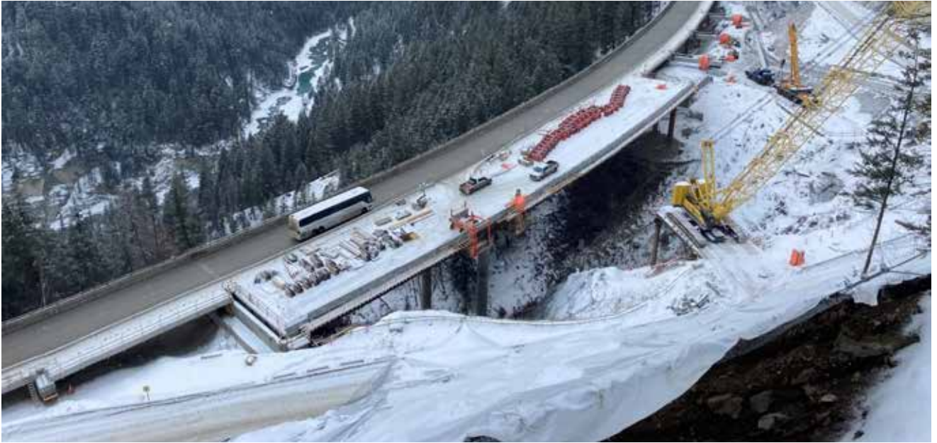
PHOTO 1. THE PARTIALLY COMPLETED BLACKWALL BRIDGE THROUGH THE TABLE MOUNTAIN AVALANCHE HAZARD AREA. THE OLD HIGHWAY GRADE CAN BE OBSERVED ADJACENT TO THE SLOPE. THE NEW FOUR-LANE BRIDGE WILL ALLOW LARGE AVALANCHES TO PASS UNDER THE HIGHWAY TO REDUCE THE HAZARD.
