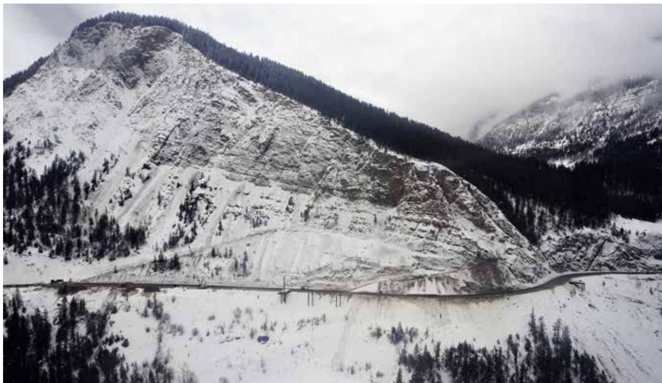
FIGURE 1. LOCATION OF PHASE 4 OF THE KICKING HORSE CANYON PROJECT (KHCP4) IN RELATION TO THE PREVIOUSLY COMPLETED PHASES 1 THROUGH 3 CONSTRUCTION PROJECTS. CREDIT: BC MOTI IMAGE HTTPS://WWW.KICKINGHORSECANYON.CA/ABOUT/PROJECT-OVERVIEW/
