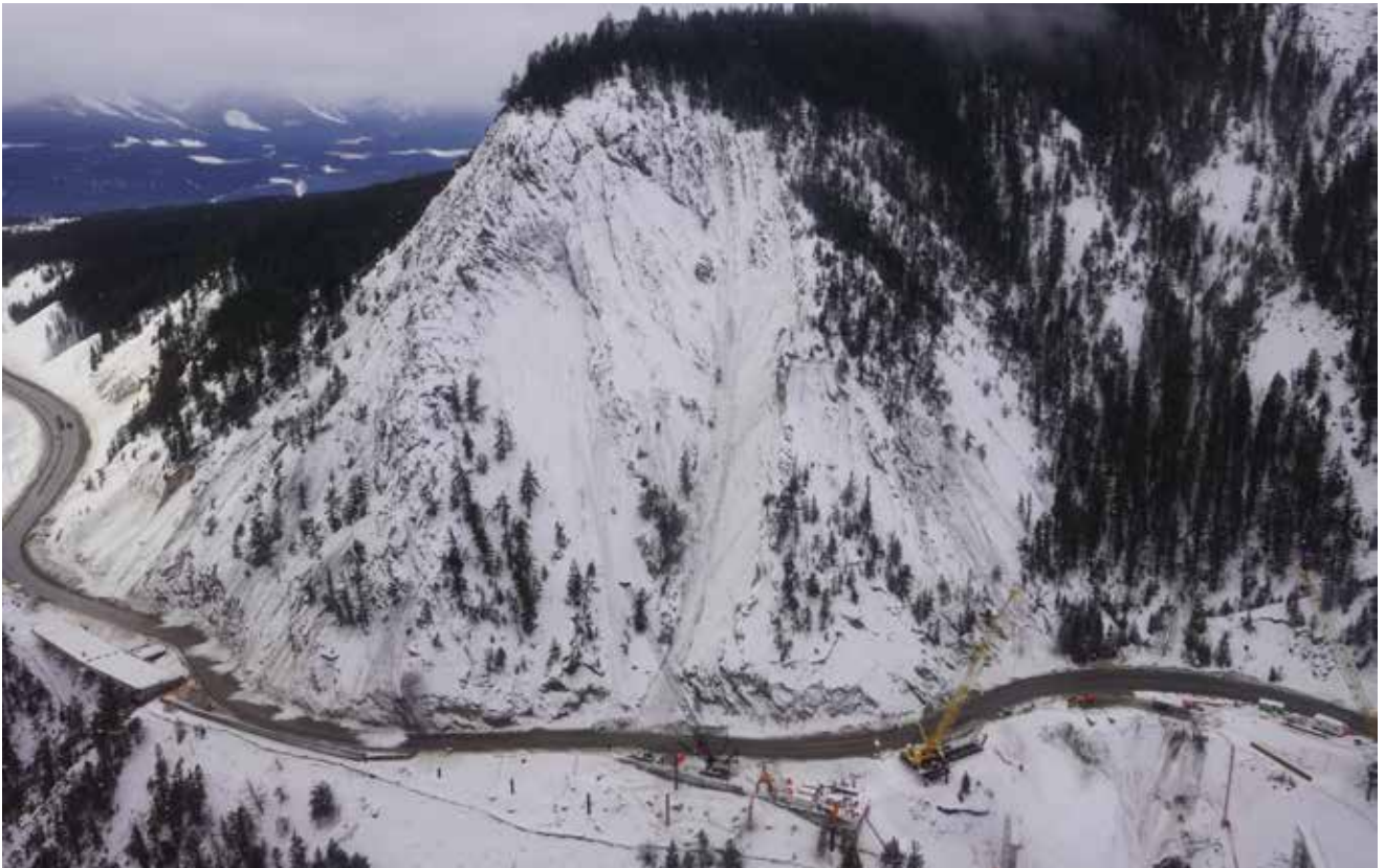
PHOTO 2. AVALANCHE PATH 4.8 AT THE WEST END OF PHASE 4 CLEARLY SHOWS RISK TO THE HIGHWAY AND A WORKSITE. THE CPKC TRACK IS LOCATED IMMEDIATELY DOWNSLOPE OF THE WORKSITE.
