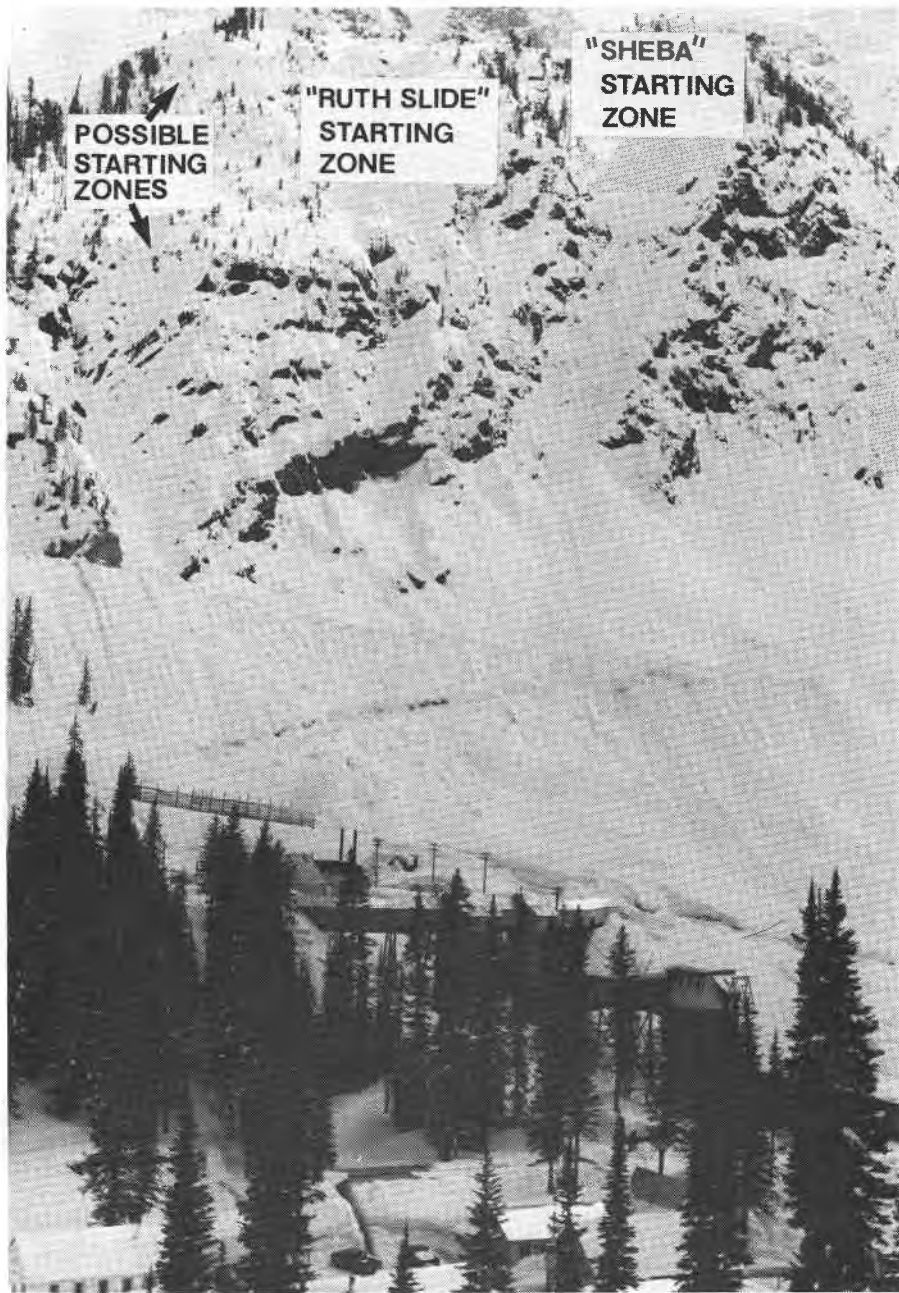
Figure 17 Ruth-Vermont Mine, showing Ruth (left) and Sheba (right) avalanche paths; the powerhouse is the uppermost building. An avalanche-catching barrier was later built.
