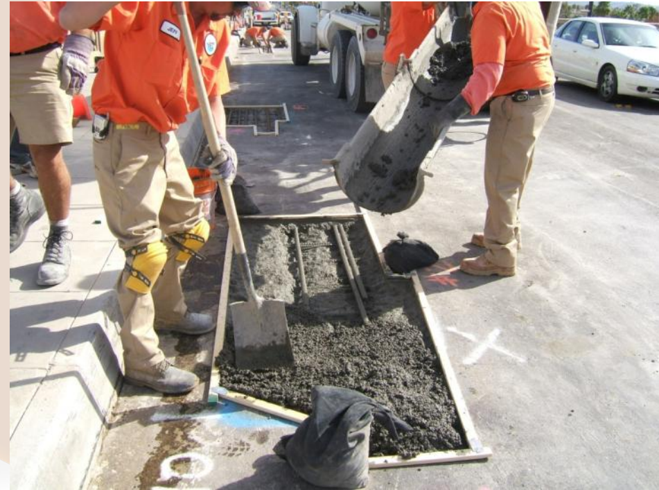
Forming edges and placement of microsilica concrete to protect reinforcing steel
