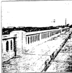
The hand rail and sidewalk on the new bridge adds beauty to the bridge, and safety for pedestrians.
