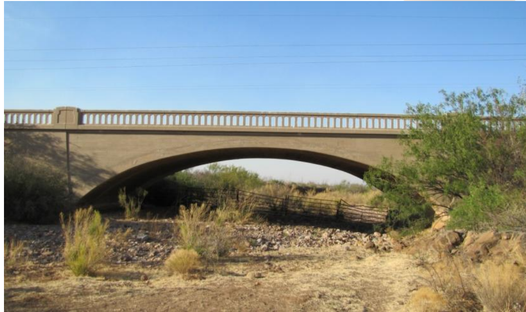
US 80 Lowell Arch Bridge
