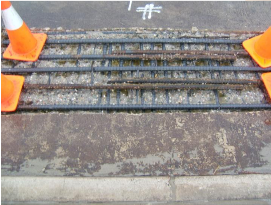
Removal of deteriorated concrete
