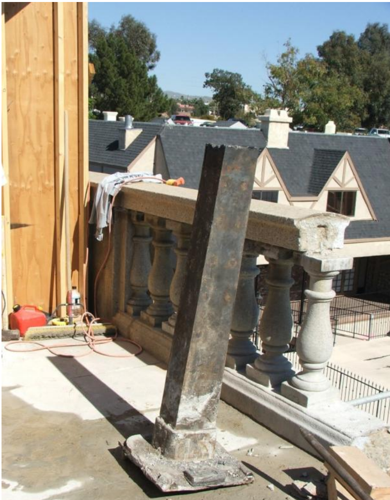
Remove rusted lamp support post
