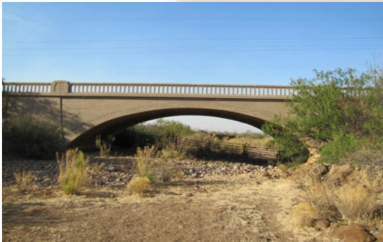
Lowell Arch Bridge (1911)
