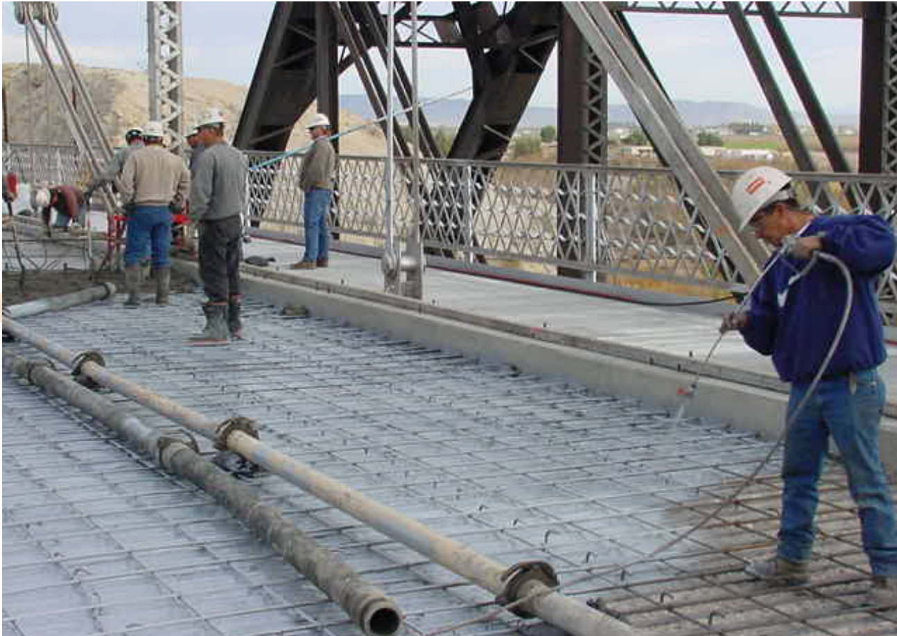
Bridge Deck Construction
