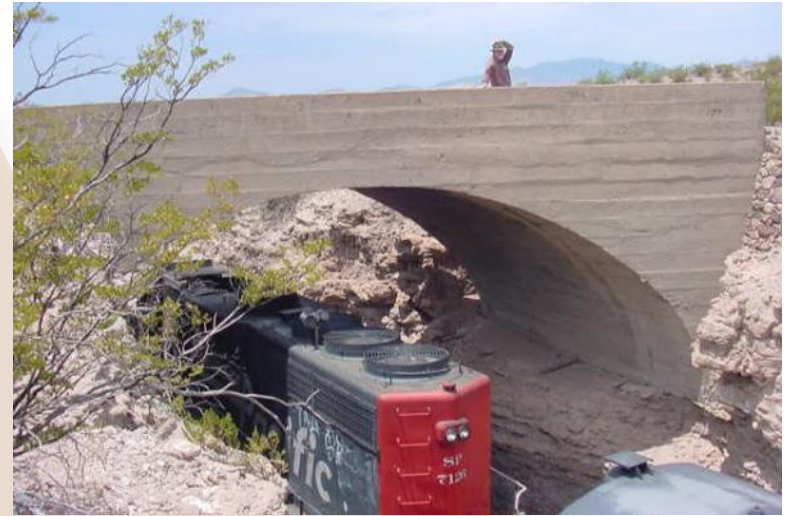
Solomonville Road Overpass (1907)
