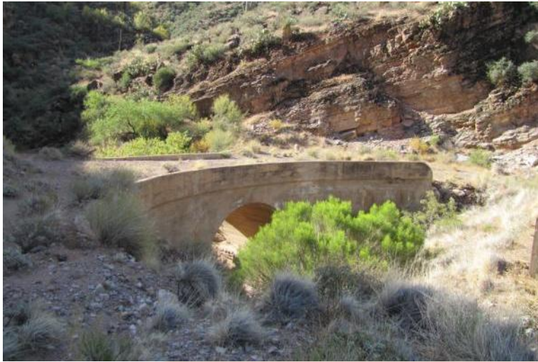
Alchesay Canyon Bridge (1905)
