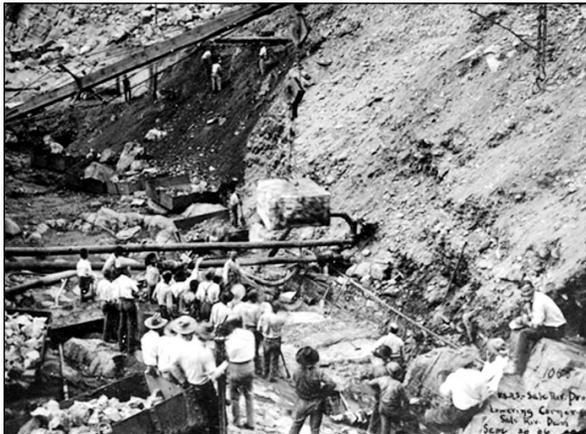
*Crews lowered the first stone at Roosevelt Dam on September 20, 1906. This cornerstone sits on the bedrock of the Salt River and established a firm footing for the Salt River Project.*
