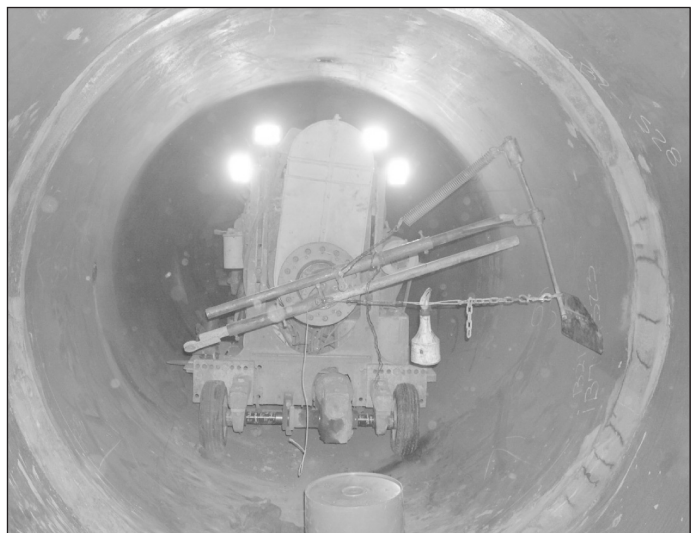
Figure 4 – Mortar Troweling
