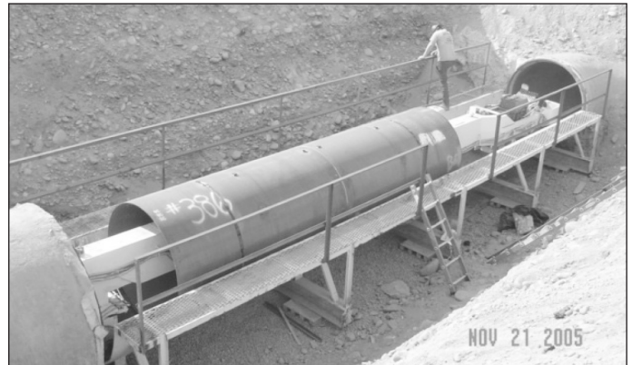
Figure 2 – Cradle with Collapsed Liner Ready for Installation
