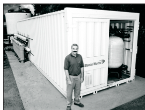
California Water Service Company 1100 GPM Nitrate Removal Unit Jim Luongo – Superintendent of Production
