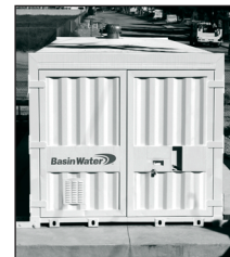
City of Pomona 1000 GPM Nitrate Removal Unit
