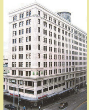
1970s Securities Building
