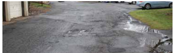
(above) ROADS — Spot asphalt repairs and deferred maintenance can cause base and sub-grade deterioration and greatly increase road replacement costs.
