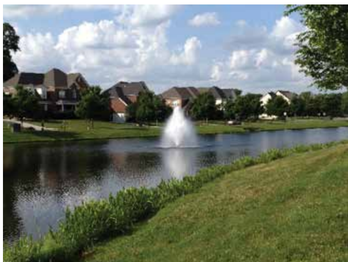
(above) Floating fountain aerators provide effective oxygenation in shallow lakes and ponds, which can help reduce undesirable algae by facilitating the conversion of phosphorus to forms that do not sustain algae growth.
