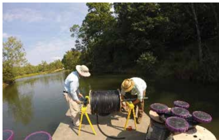
(above) A submersed aeration system can help oxygenate the water column in deeper lakes and ponds. These systems improve vertical mixing at depths where water is not naturally stratified by using an on-shore compressor to pump oxygen to the bottom of the waterbody.
