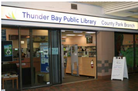
County Park Branch Library
