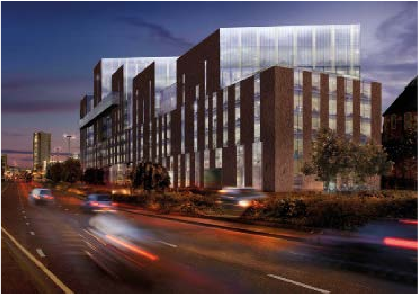
One of the largest construction sites in Europe will give rise to Ulster University's new campus at Cathedral Square, Belfast.
