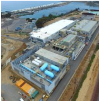
Carlsbad Seawater Desalination $1 billion
