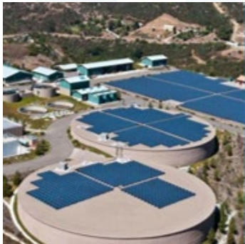
Twin Oaks Valley Water Treatment Plant $179 million
