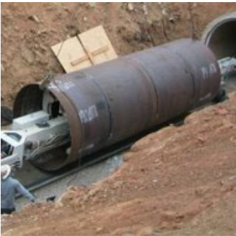
Pipeline Relining $493 million
