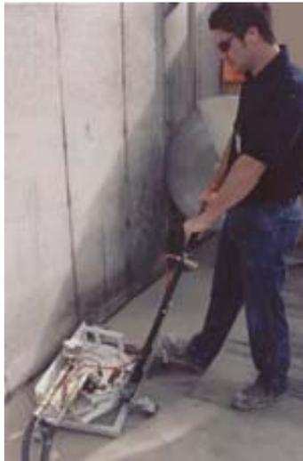
**For making the flush cut along the floor, a flush cut hand saw on a cart could be used instead of a flush cut wall saw.**
