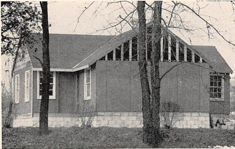
Construction—December, 1950 (Photo, Sqdn-Ldr. J. T. L. Lowe.)
