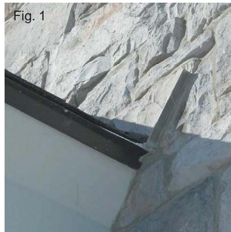
We also need to be concerned with areas where water channels and creates a dam. In these areas higher step flashing and/or a cricket may be installed. It is common to see this problem on the back side of a chimney.
