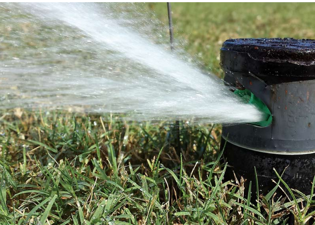
Fig. 6 The selection of the right sprinkler head nozzle can make a big difference in irrigation flow and system efficiency. Changing from dark green #23 nozzles to light green #10 nozzles shown here would reduce flow from 23.9 gpm to 10.3 gpm, per head. Although this would reduce the radius of coverage, it would also reduce the total flow, which would reduce the pressure loss due to friction in the pipes.
