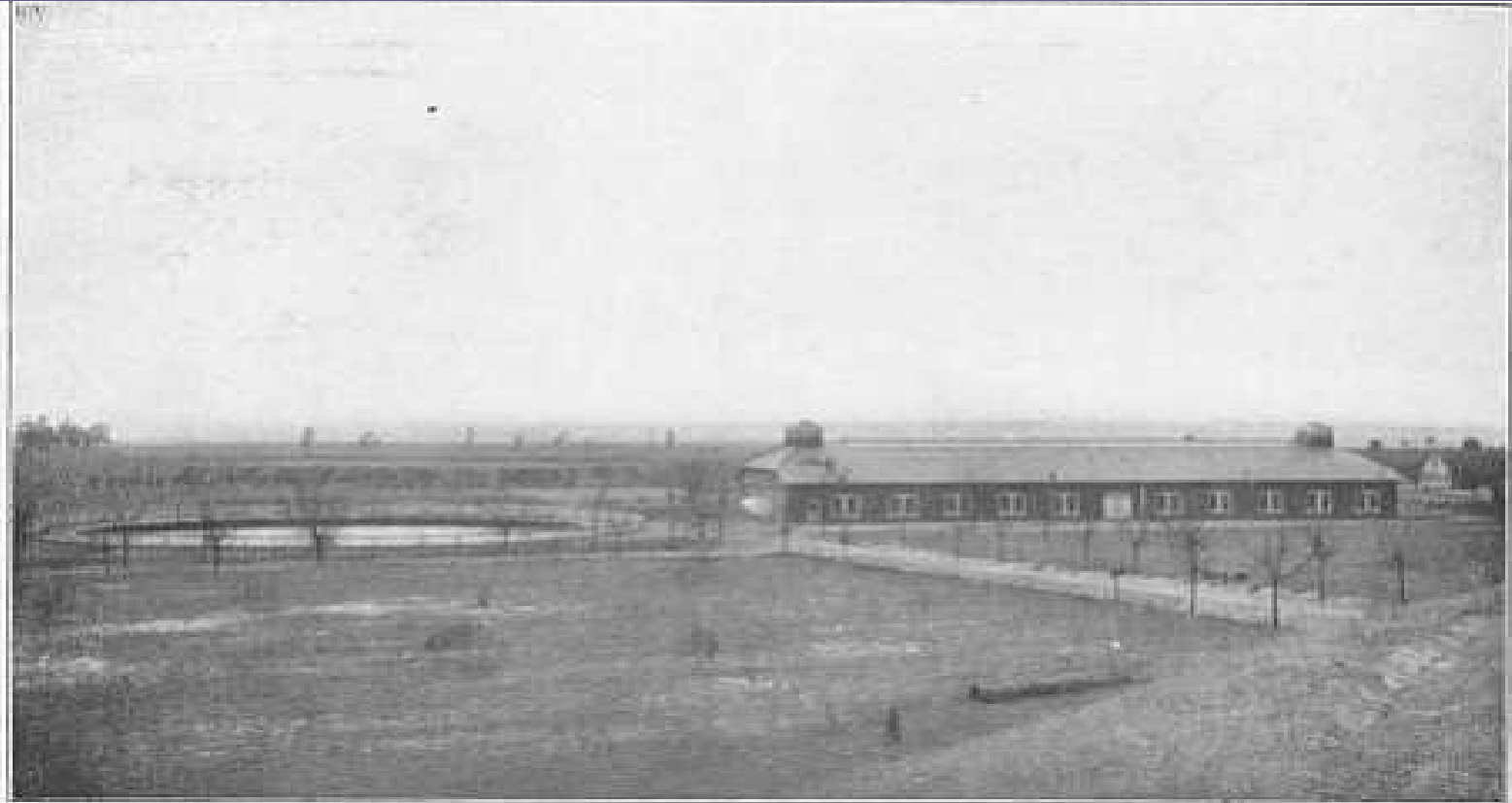
First Filter Plant on Highland Avenue
