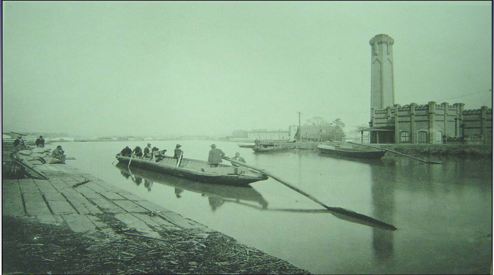
Canal Basin & 1884 Pump House
