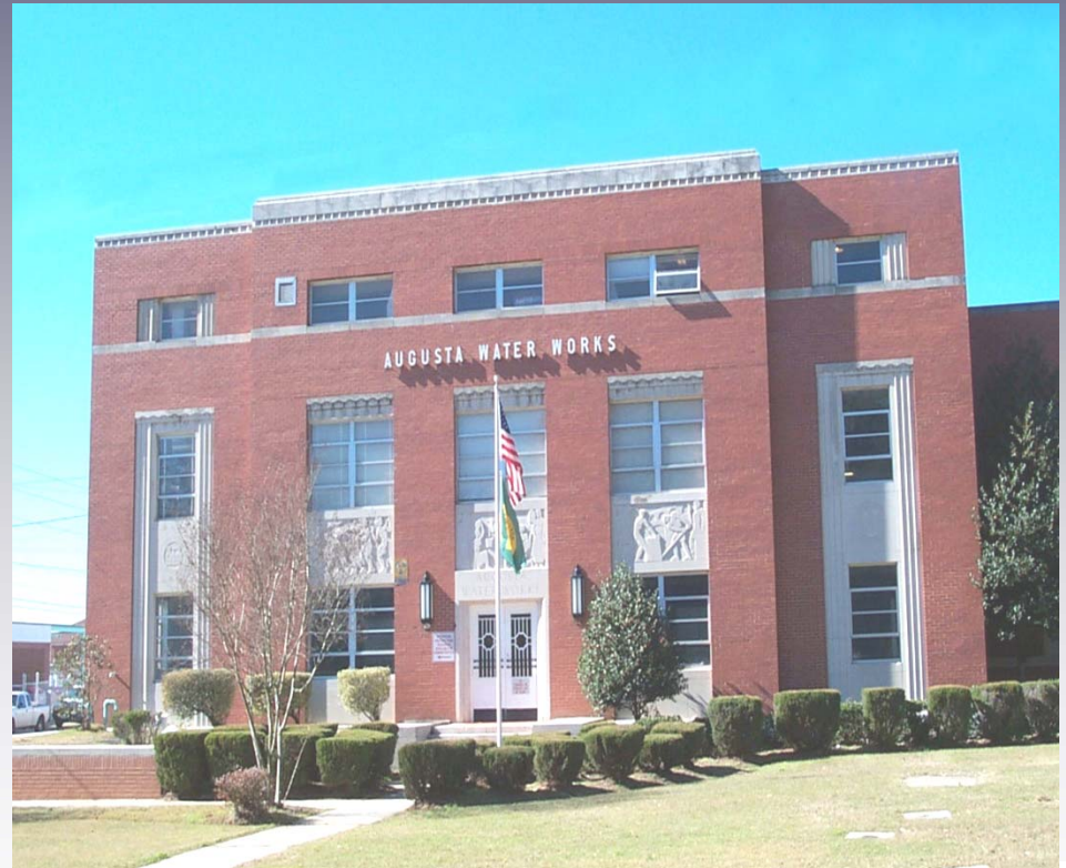
Filter Plant on Highland Avenue
