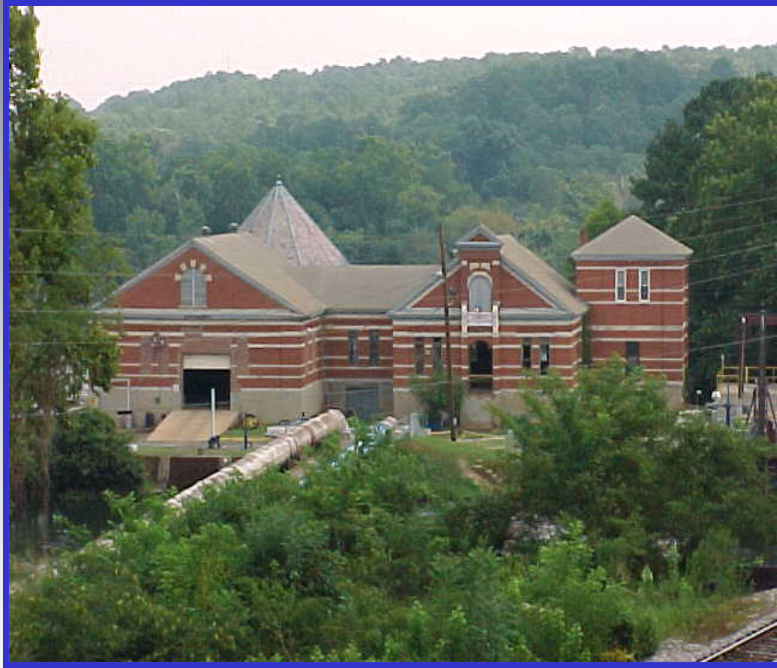
Goodrich St. Pumping Station
