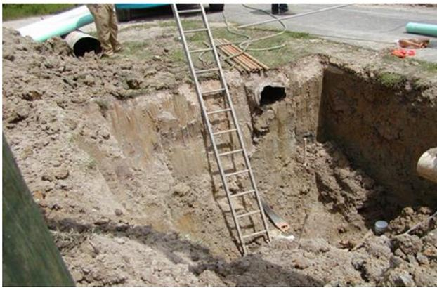
Excavation 8' deep, 12' long, 11' wide with vertical walls. Employees were boring under the roadbed to install a 6" sewer line tap on south end of trench.
