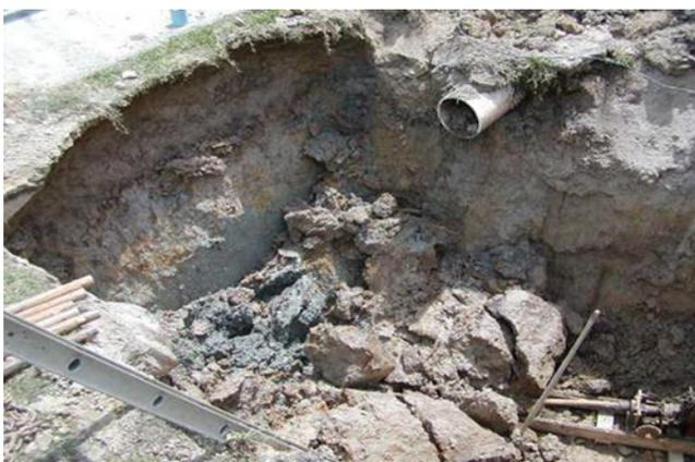
Wall collapses. The portion of the wall that fell was 15" wide by 9' long by 5' deep. Weight of the dirt was calculated to be 6,187 pounds... just over 3 tons.
