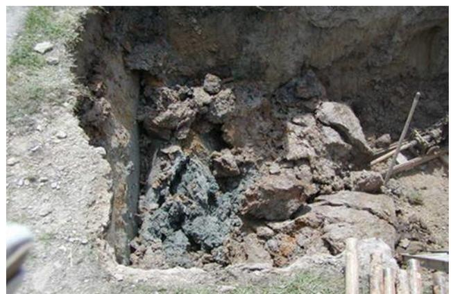
It took 26 seconds from the appearance of the fissure to the collapse of the wall. The employees would have been struck-by the collapsed wall while installing the sewer line.
