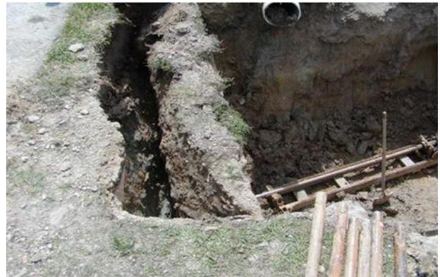
The ground surface/wall on the road side of the trench collapsing. Time : 1:06:16 PM.
