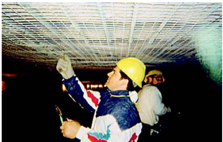
Fig. 7: Placing 2 in. x 2 in. galvanized welded wire fabric over reinforcing to aid in build-up of shotcrete material and to make the repair monolithic with the substrate
