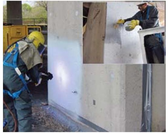
*Fig. 6: Activated arc-sprayed zinc metalizing providing cathodic protection on bridge substructure*
