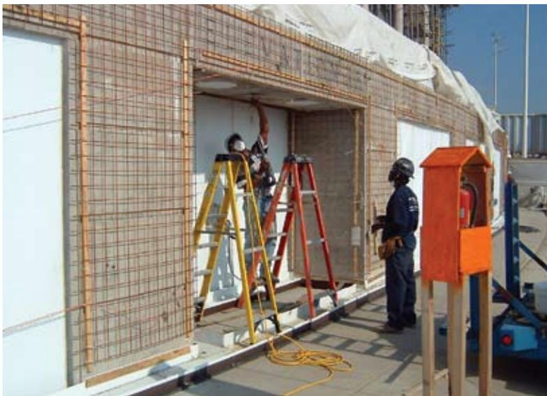
*Fig. 1: Electrochemical realkalization of carbonated concrete façade on airport terminal building*
