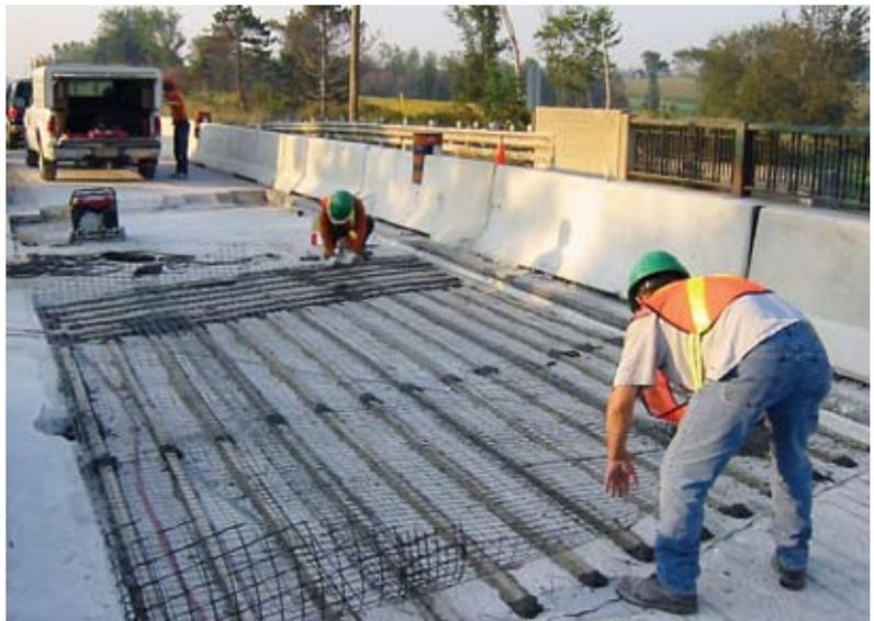
Fig. 3: Galvanic anodes used in bridge deck overlay system
