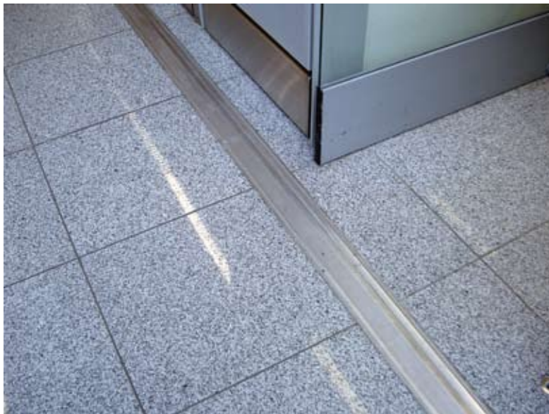
Interior joints in high-point load stadium environment
