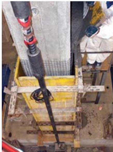
Fig. 5: High-performance jacket casting
