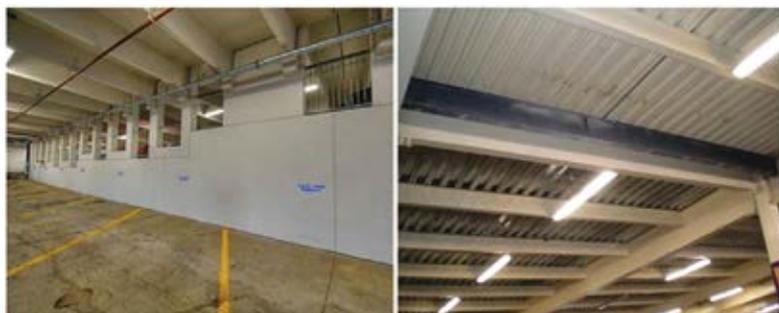
(c) Precast double tee beams and precast light walls (d) Steel frame with concrete on metal deck
