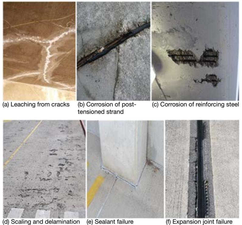
Fig. 3: Common types of deterioration in parking structures
