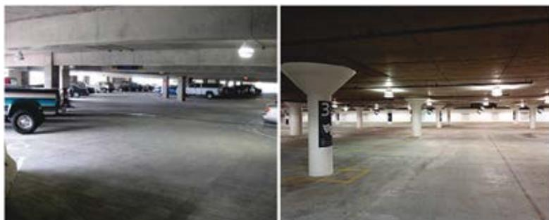
(a) Cast-in-place long span post-tensioned (b) Cast-in-place flat slab post-tensioned
