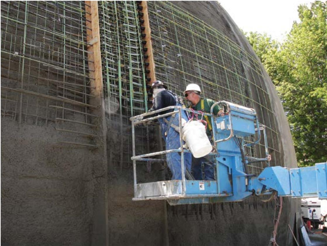
Fig. 2: Wet-mix shotcrete installation at dome structure
