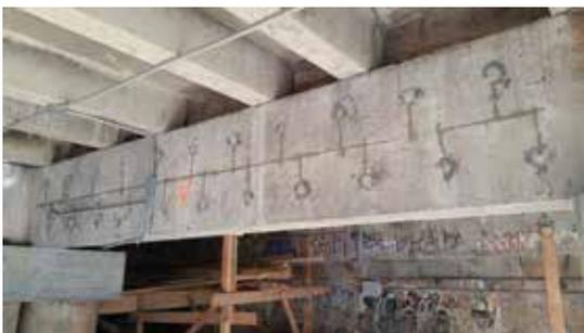
Despite previous repairs, the structure continued to degrade over time. After a comprehensive analysis, impressed current cathodic protection was selected to provide long term protection to the corroding chloride-contaminated concrete beams.
