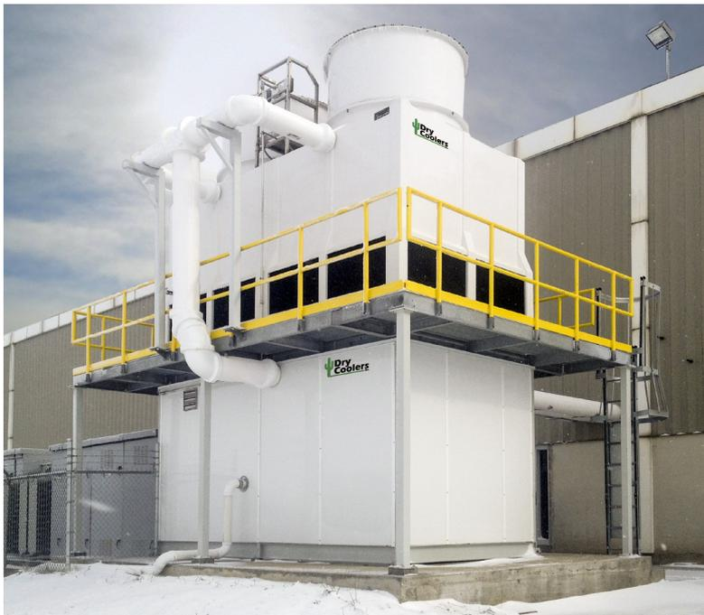
Pictured is an evaporative closed-loop cooling system for multiple vacuum furnaces. 3D computer modeling allows Dry Coolers to produce the most compact and practical skid-mounted equipment. High-quality fabrication and optimized thermal engineering combined for a reliable and competitive system.
