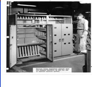
Electronics cabinet for military system that would be delivered by air. All magnesium sheet and extrusions. 1960's
