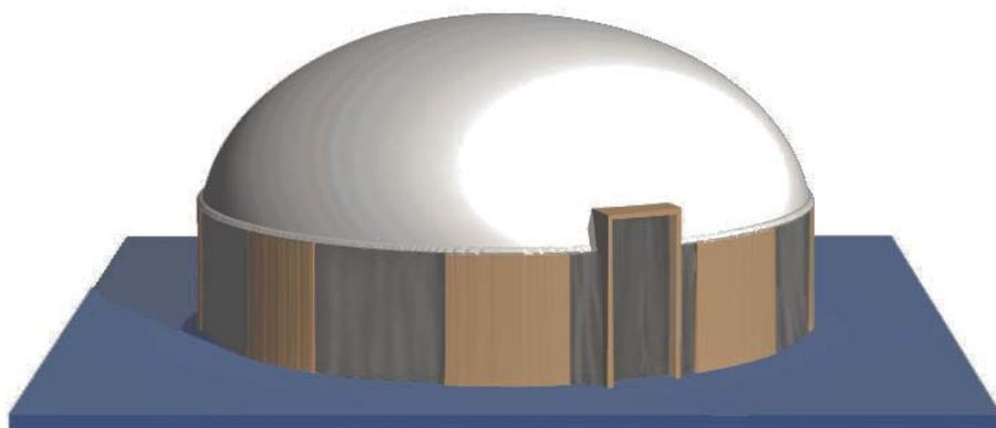
**This graphic by Observatory artist Chris Butler (which was prepared for the bid package) shows the flattened shape of the dome and the structure of the walls where solid panels alternate with curtains. As constructed, curtains surround the entire exterior.**
