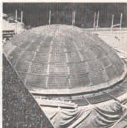
Rod reinforcement and paper-backed wire mesh
