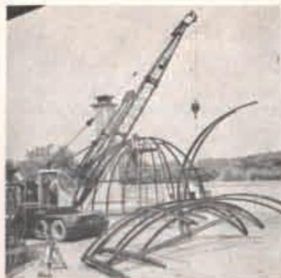
Site steel assembly; prefabricated base and ribs
