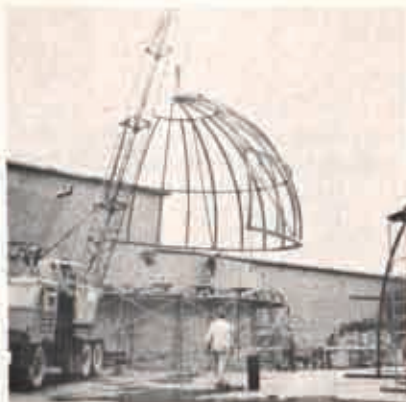
Lift of one-half assembly
