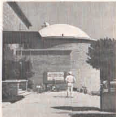
Integral float finish for appearance and sealing
