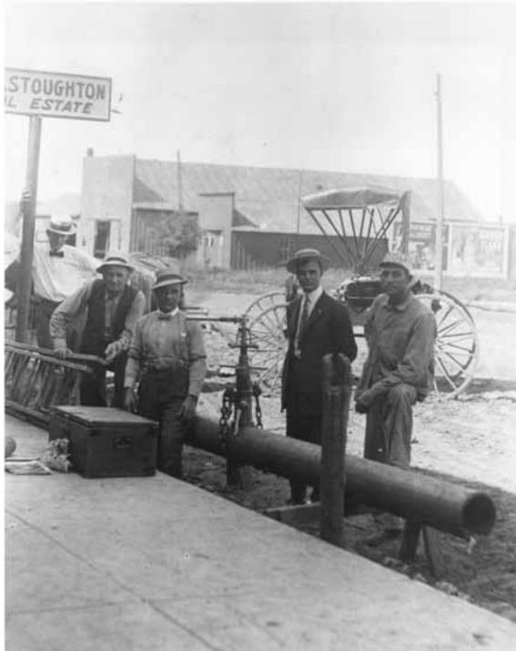
A demonstration of an early Mueller® B Tapping Machine
