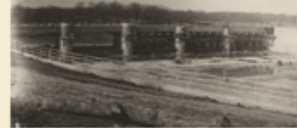
Spaulding Dam construction, 1934
