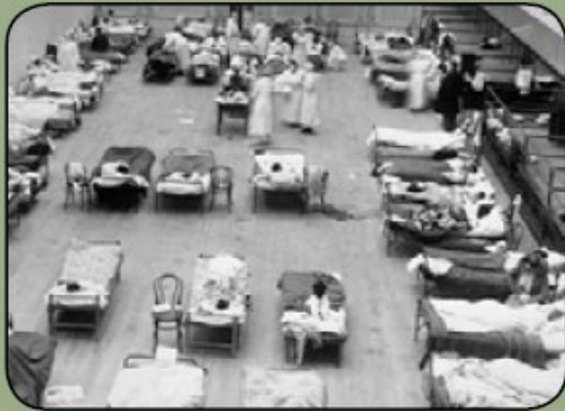
The Oakland Municipal Auditorium in use as a temporary hospital during the 1918 flu epidemic.
