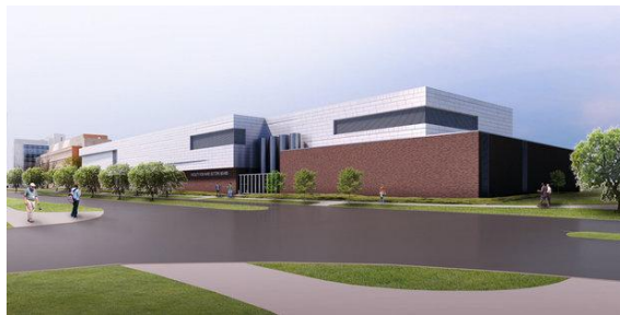
The 220,000 sq. ft. Facility for Rare Isotope Beams is under construction on the MSU campus. This scientific facility is anticipated to create over $1 billion in economic activity in Michigan.
