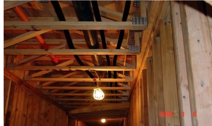
Over Ceiling Joists/
