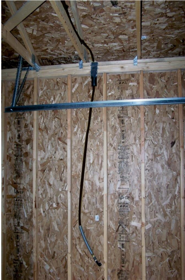
Striker Plates and Floppy Installed
