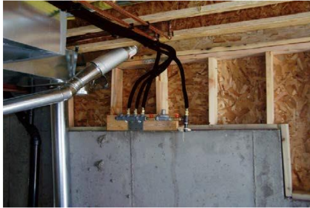
Beneath Floor Joists
