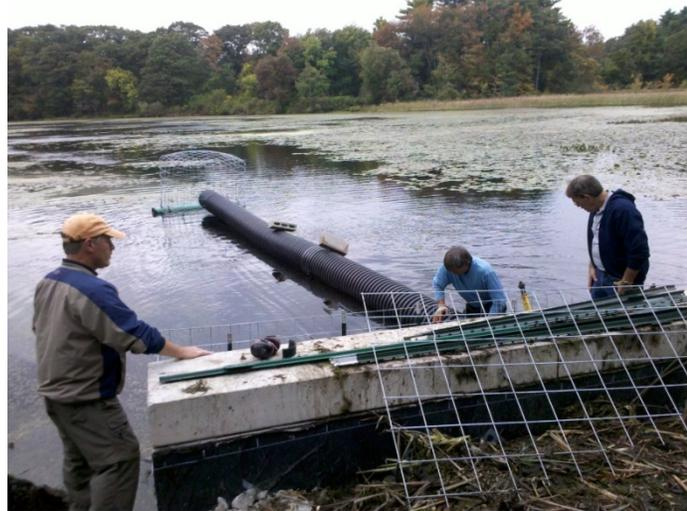
Even though the beavers can dam against the fence and hold back some water, the pipe will allow water to move freely in and out of the pond through the installed pipe. It is normal for the fence surrounding the spillway to collect some debris. Beaver Solutions conducts seasonal site visits to remove significant obstructions.
