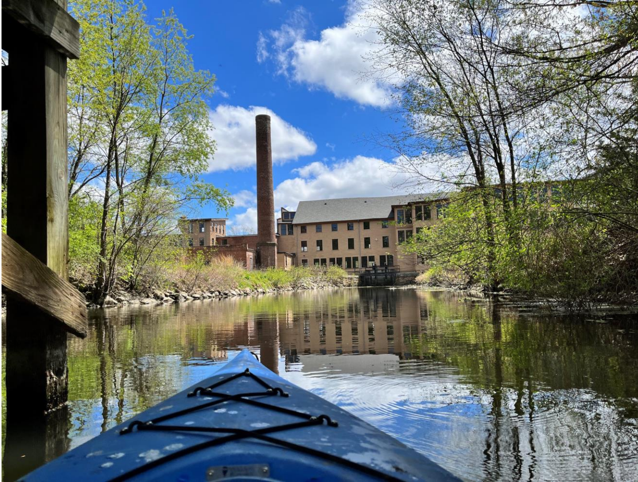
Blackstone Canal, looking toward the Stanley Woolen Mill
