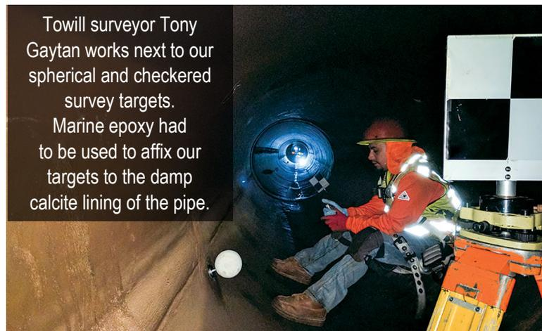
Towill surveyor Tony Gaytan works next to our spherical and checkered survey targets. Marine epoxy had to be used to affix our targets to the damp calcite lining of the pipe.
