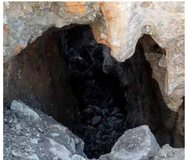
**Several of the holes close to the South Sprigg Street Bridge caused the paved creek bank to fall in, and also caused the road pavement on the north end approach to cave in.**
