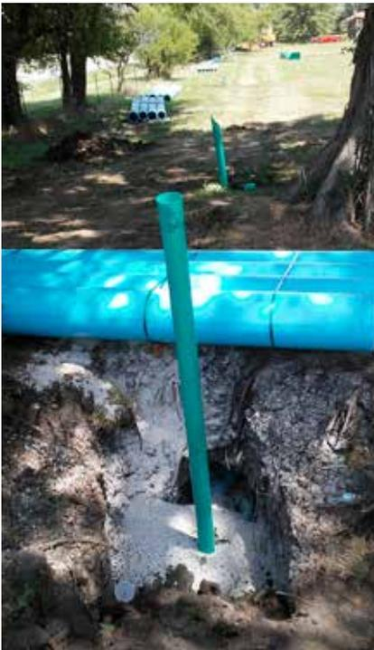
**To reduce the construction disturbance to the community and its residents, the pipe line was bored in lieu of open-trench cut and installation at many locations along the transmission main alignment. This saved numerous trees and landscaping items.**
