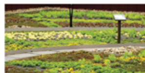
Extensive Vegetated Roofing System
